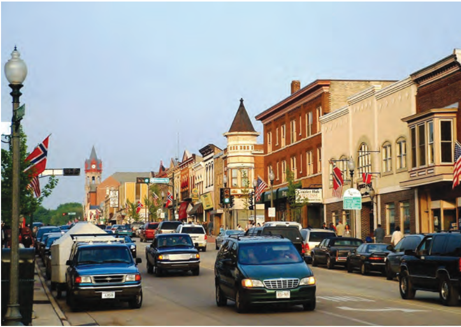
Stoughton's restored and lively Main Street. The Façade Improvement Program offered matching grants to any building owner willing to refurbish their storefront.
