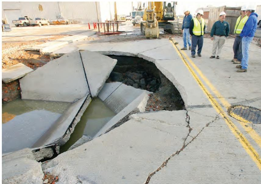
*A water main break in Gillette, Wyo. in August 2006. About 3 million gallons of water erupted causing at least \$100,000 in repairs and requiring traffic diversions.*
