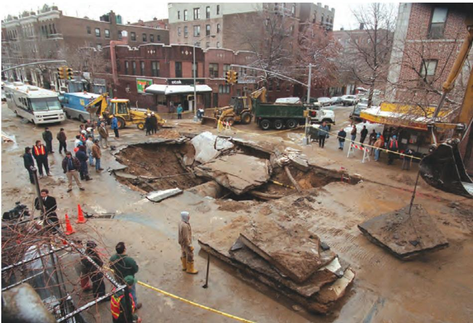
*Emergency construction crews examine a ruptured water main in the Queens Borough of New York January 3, 1996.*
